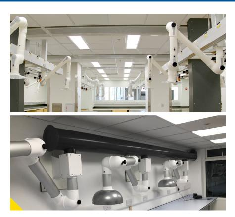
As an installer of LEV extraction arm systems, The Fume Cupboard Company is your trusted partner for seamless installation and reliable maintenance services, catering for wall, bench, and ceiling-mounted fume extraction arms.
